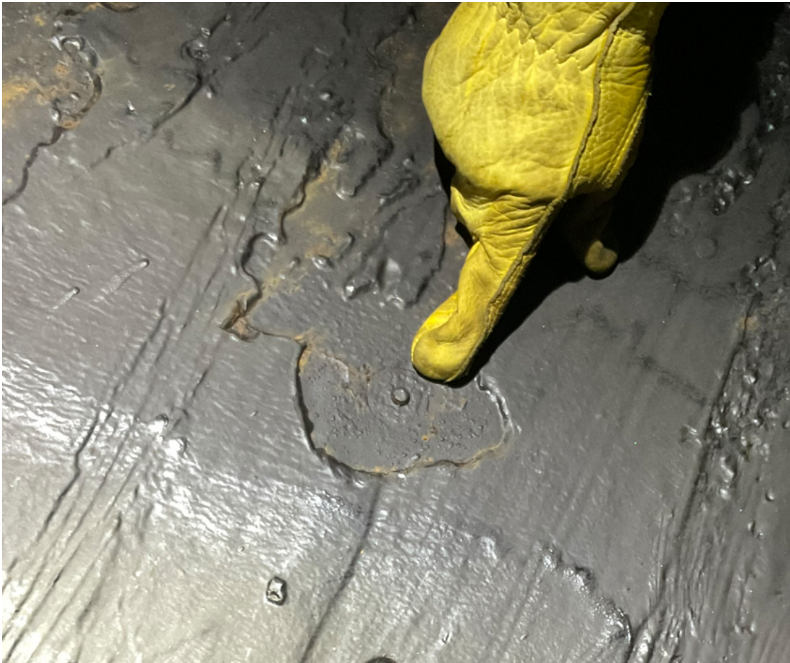
Figure 4.—Example of a pressure tap that has been covered by a repair coating.
